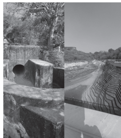
The water regulating well (left) with an anti-clockwise direction ramp used to control water speed and the reservoir (right) cut into the rocky terrain which can store nearly 40 million litres of water.
